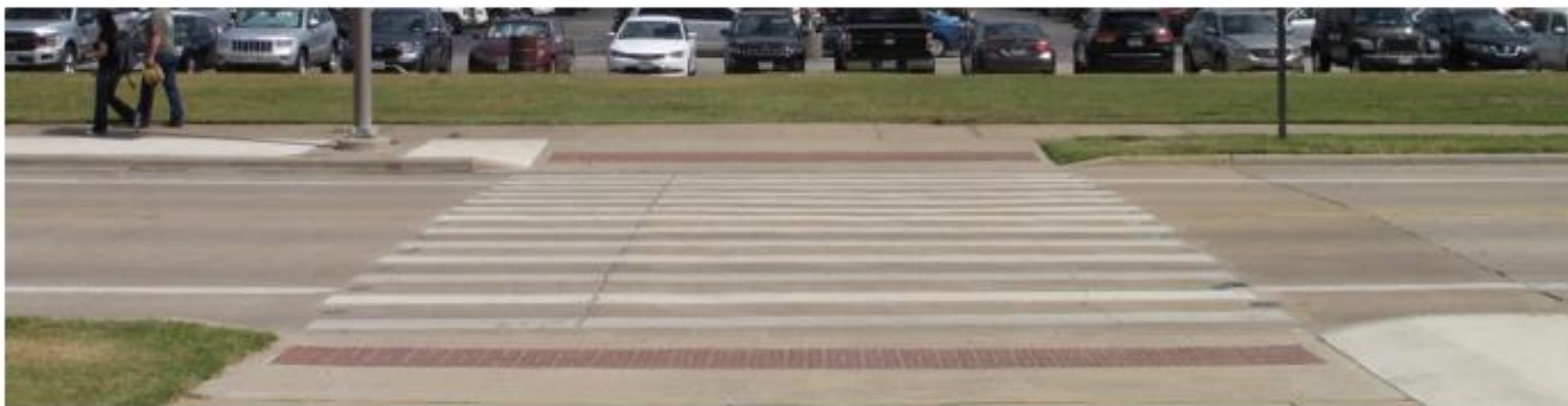
Figure 92: Walkway at PEAP across Penberthy Boulevard
